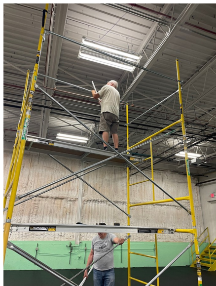
Carl on scaffolding, working maintenance at the club
